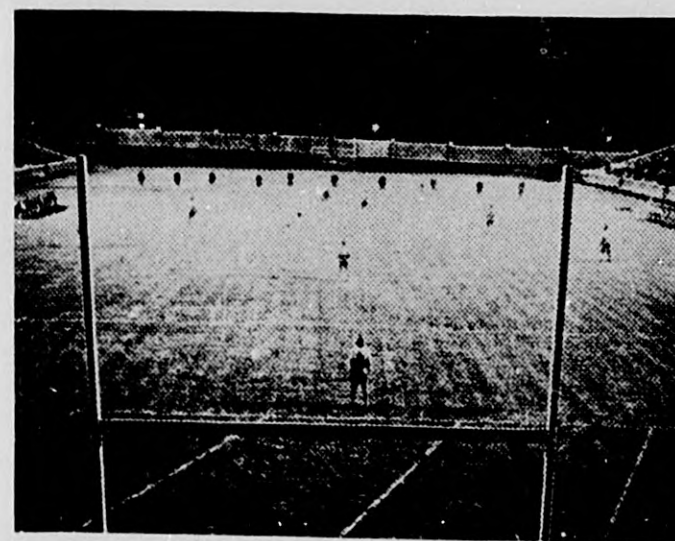
Night photograph of Temple Stadium, Philadelphia, Pennsylvania, floodlighted with G-E projectors
