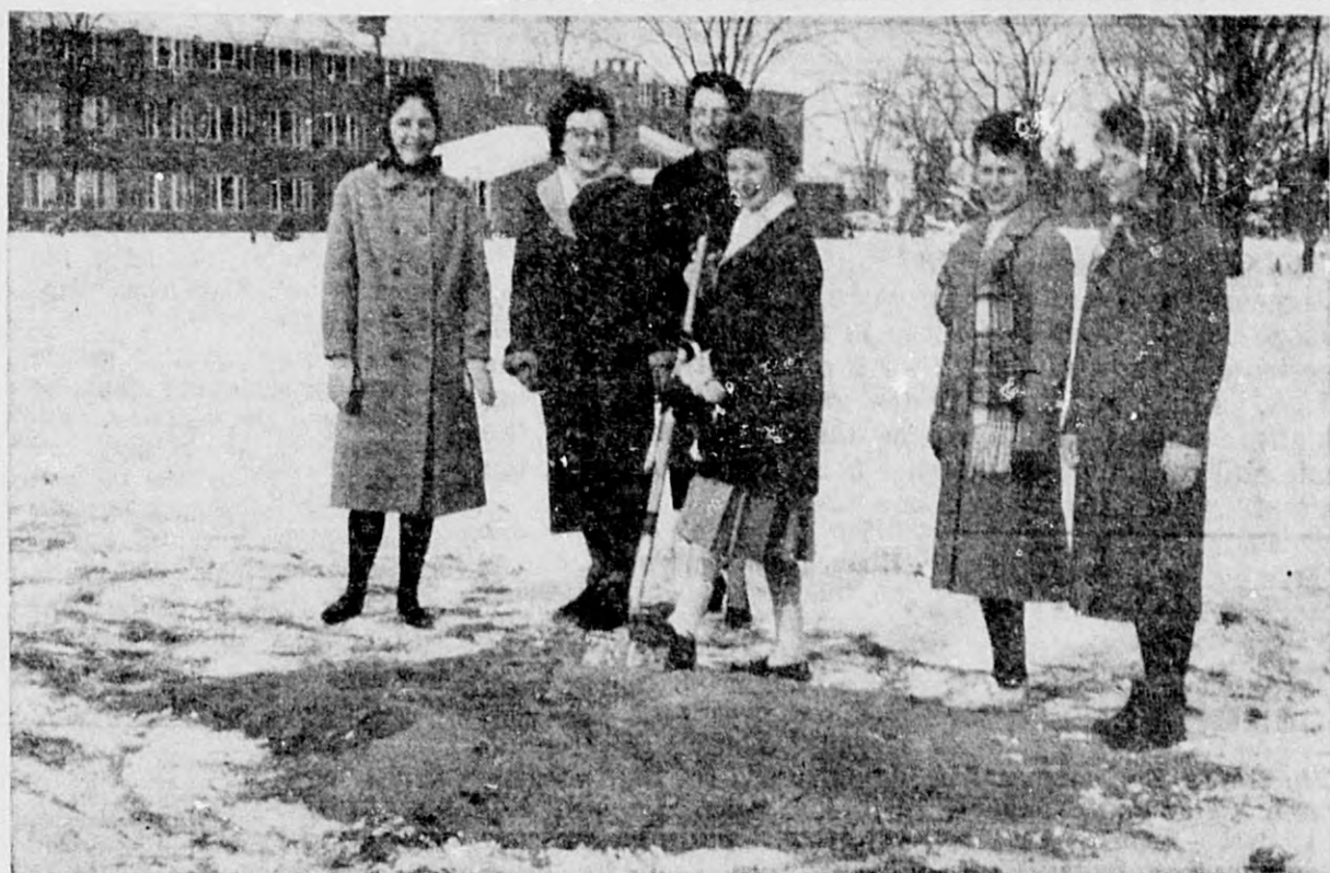
In spite of the weather, ground was broken January 27 and workmen started construction almost immediately on the new women's residence hall located behind Mary Gelston Hall.
