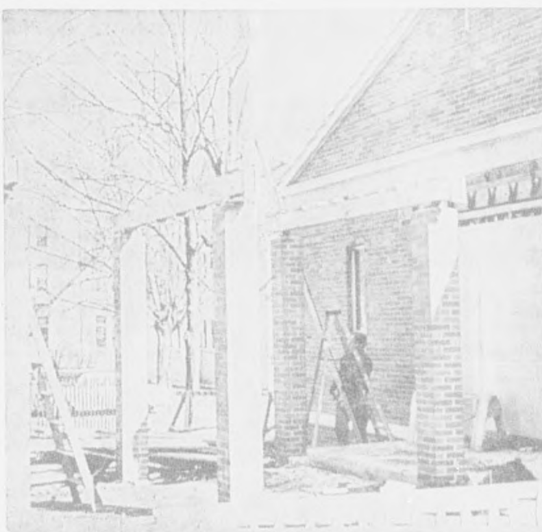
The fenced-off construction work at the north end of the Reid-Knox Administration Building is to become an extension of the Reid-Knox building, a 20 by 24 foot pit in which telephone equipment will be housed. The structure will be mainly below ground, with a lobby over the pit, for dryness. The only cost to the college will be that of constructing the building to house the installations. Dr. Stephen Meyer, business manager of the College, estimates that this addition will cost $15,000. He emphasizes also that this installation will be an improvement to all telephone services on campus. (Photo by Jacobs.)
