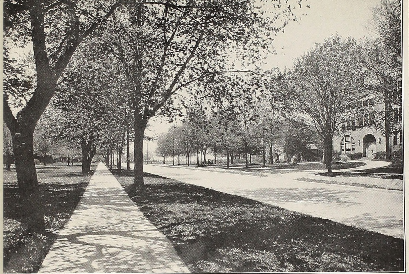
Looking West on Superior Street
