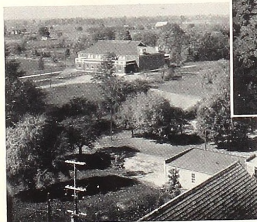
View towards Memorial Gymnasium from Admin- istration Building.
