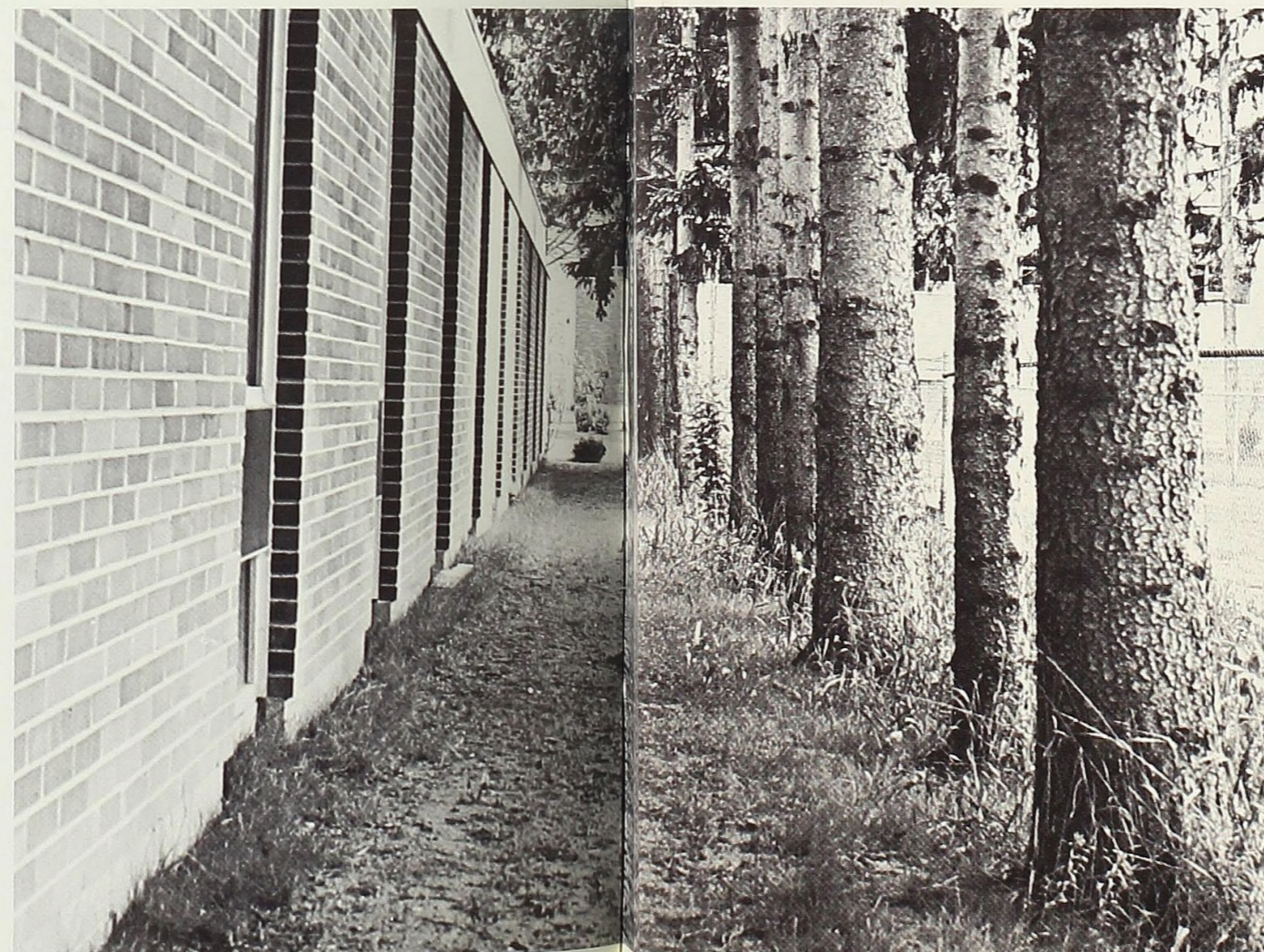
New Office Building
