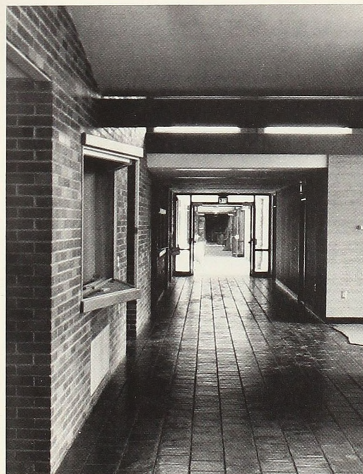
The newly tiled hallway connects the entire building.
