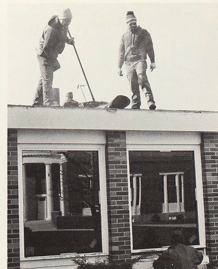
On warmer winter days, the workers replaced the roof and windows.
